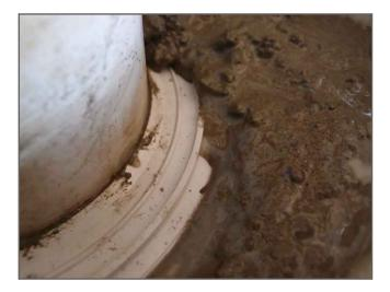
Sx Termite collars key strongly into the concrete to block termite access.
