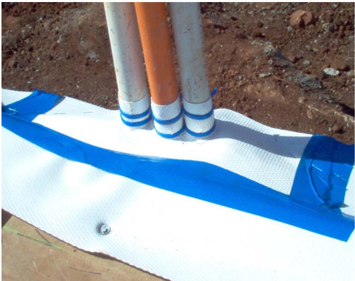
Above: Multiple penetrations in the perimeter cavity using HomeGuard DPC
